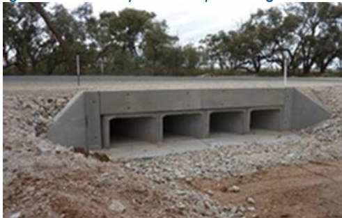
Figure 5-3 - Example multi-span bridge/culverts
